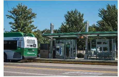
BRT Station Rehabilitation: $1,982,195
