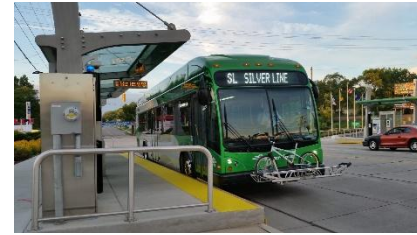
Silver Line Security Equipment: $235,000
